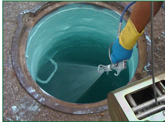
Novocoat SG2500 Lining high build epoxy application.
