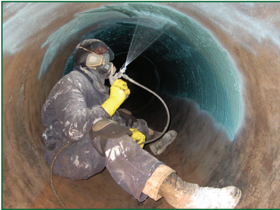
Novocoat SG2500 Lining high build epoxy application.
